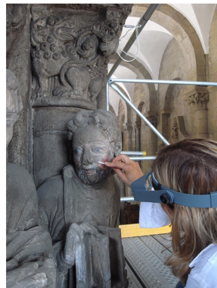
Figure 3. Surface cleaning of an apostle from the south pillar of the Portal of Glory. Cathedral of Santiago (photo: © Barrié Foundation)
